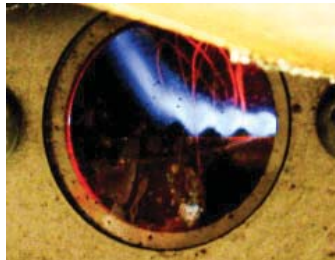
Lifting flame with too much air
