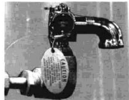
Safety valve with elbow in correct position
