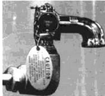
Safety valve with elbow in correct position
