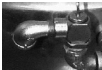
The open end of the pressure relief valve elbow must face downward.
