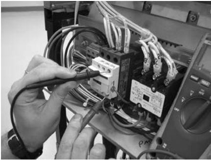
Heat contactor ohm check
