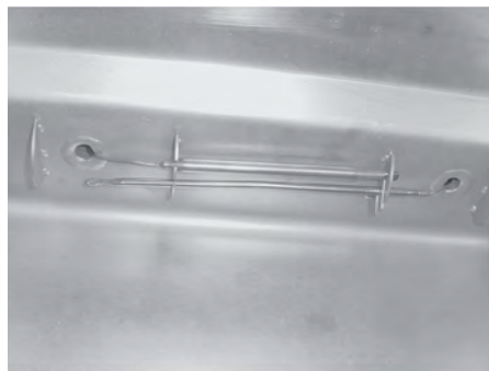
Figure 2-2 Thermostat Sensing Bulb - Gas
