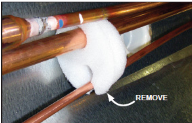
Fig. 5 Remove the shipping blocks
