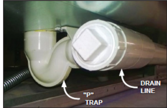
Fig. 6 "P" trap; drain line
