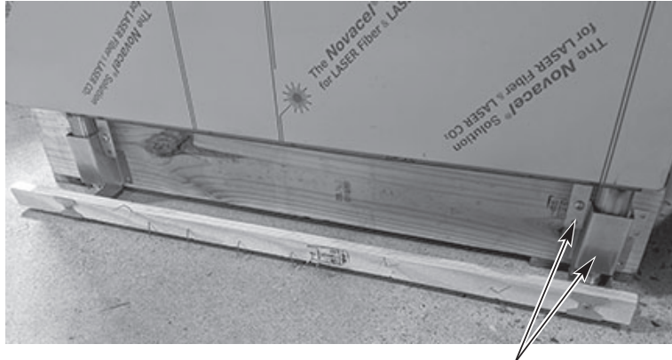
REMOVE SHIPPING BRACKETS (4 LOCATIONS)
