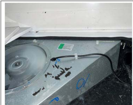
Correct – gasket is between bottom of back panel and top of fan plenum
