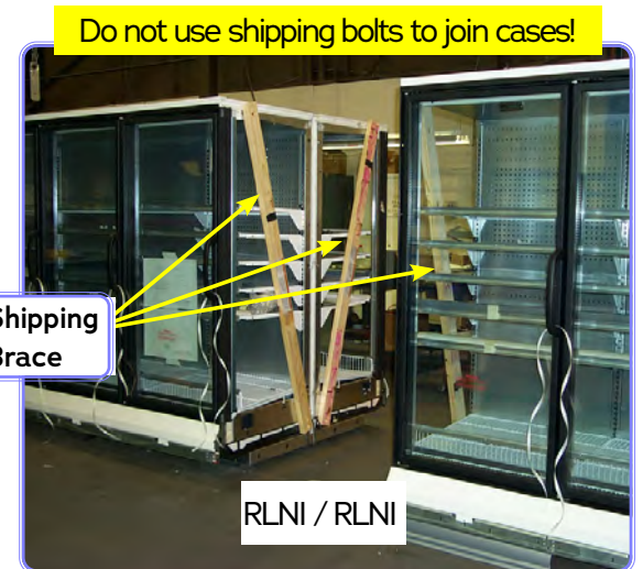
Remove Shipping Braces
