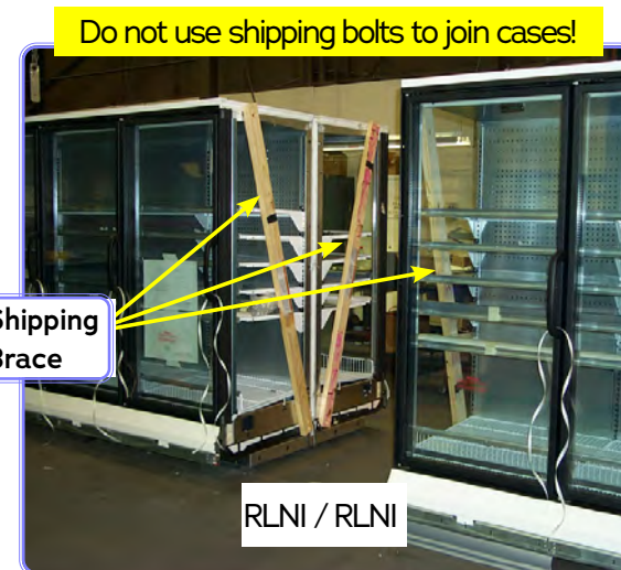
Remove Shipping Braces
