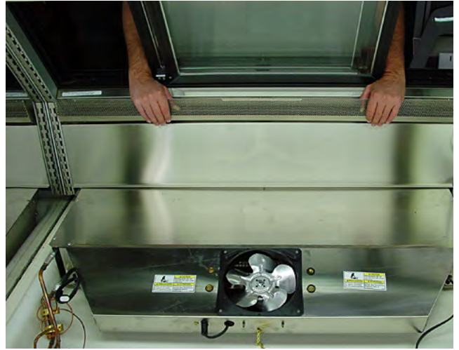
STEP 9 – Lift out upper shelf supports.
