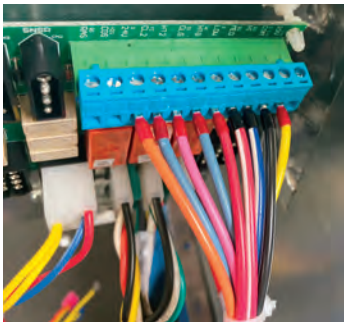
Figure 35. Mounted thermostat connection
