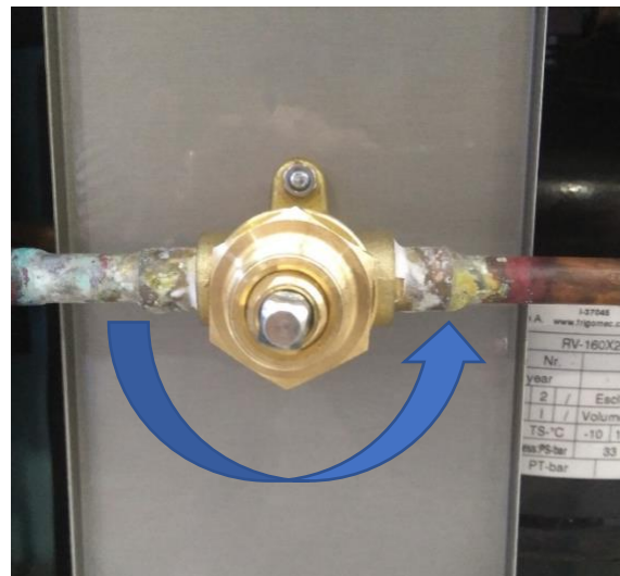
Picture 7: Turn it counterclockwise to open both taps
