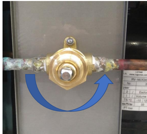
Picture 7: Turn it counterclockwise to open both taps
