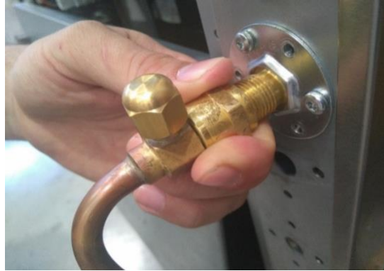
Picture 6: Thread the couplings by hand
