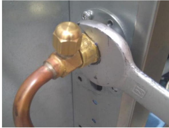
Picture 4: Tighten with a fixed wrench clockwise
