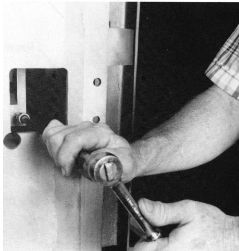
Figure 22. Using Allen Wrench to Loosen Upper Cup Crank Arm
