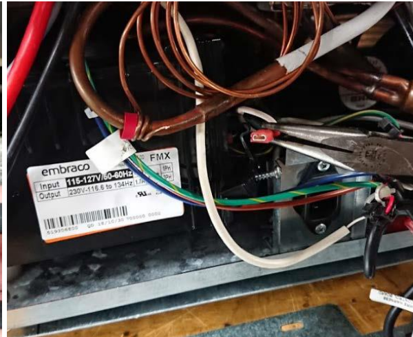
Figure 78: Ground Wire shown removed.
