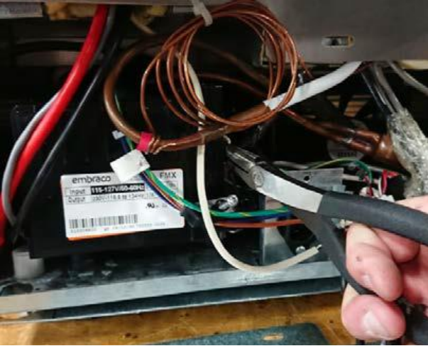
Figure 72a: Power connections being removed.
