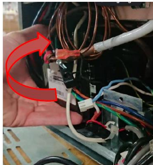
Figure 77: Inverter being removed.
