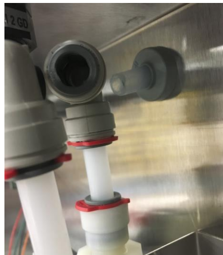
Figure L5: Controller Board Enclosure placed back in its original location.
