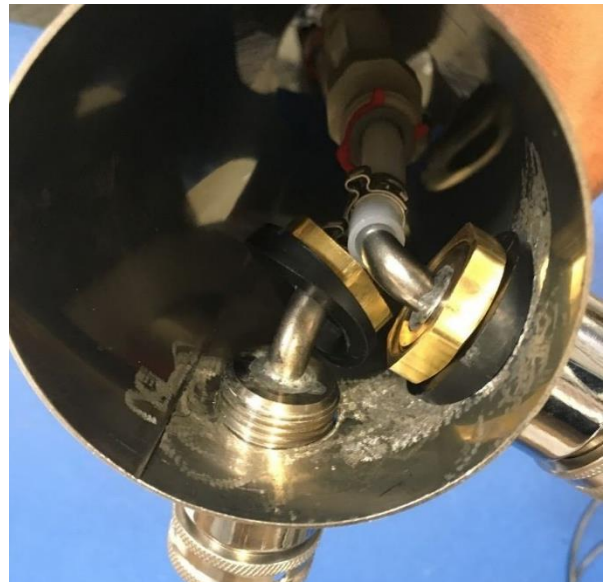
Figure H30: Threaded end of the Elbow Shank inserted through the Left Hole in the Tower.
