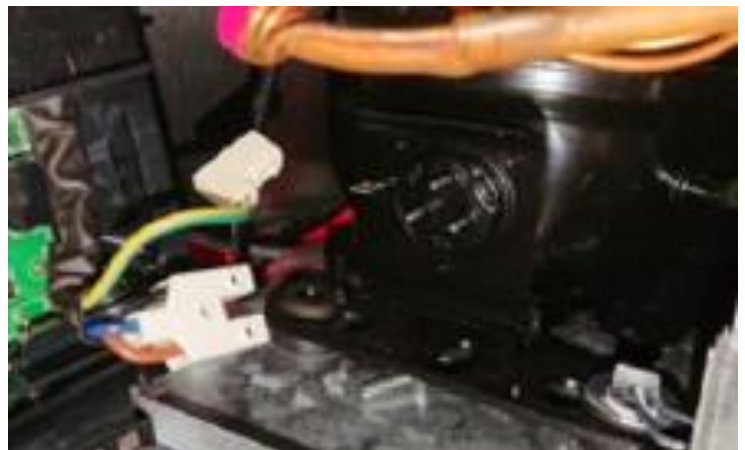
Figure 79b: Compressor connections removed.
