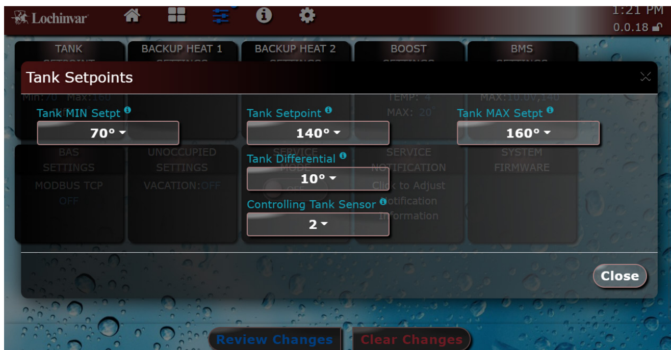
Figure 1-3 Tank Setpoints HW Screen
