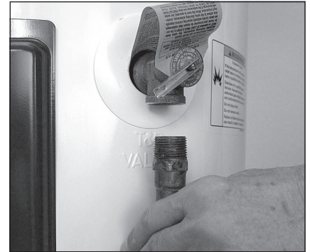
Figure 13 - Removing the T&P Relief Valve discharge pipe.
