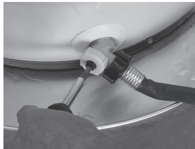
Figure 12 - Draining the old water heater.
