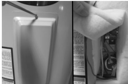
Figure 12 - Element Access Panel/ECO Compartment
