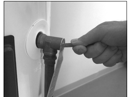
Figure 13 - T&P Relief Valve
