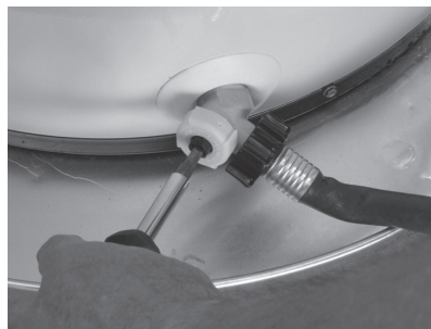
Figure 12 - Draining the old water heater.
