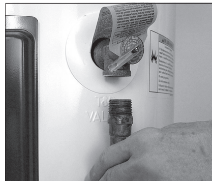
Figure 13 - Removing the T&P Relief Valve discharge pipe.
