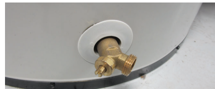
Figure 33 - Drain Valve
