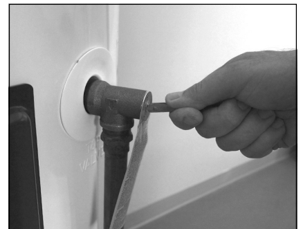
Figure 13 - T&P Relief Valve
