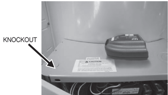
Figure 23. Knockout on Left Corner of Top Panel
