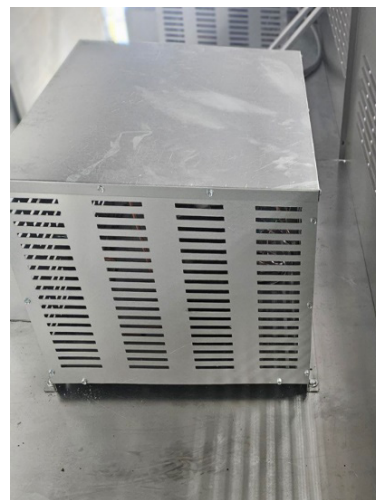
Figure 29 – Condensing unit
