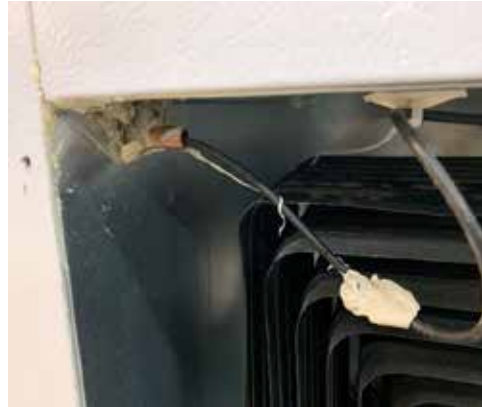
Sensor probe with bulb well foamed
