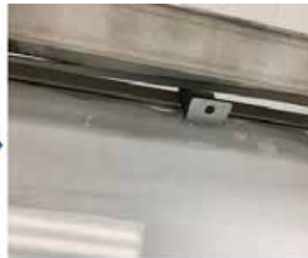
Top hinge part installation Lift the Lid to open. It will create a gap at the top and bottom of the lid. Place the top hinge as shown in the picture
