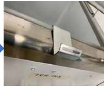
Bottom hinge part installation Place the bottom hinge on the SS top as shown in the picture above.
