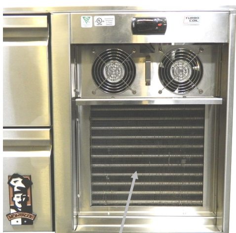
Condensing Coil
