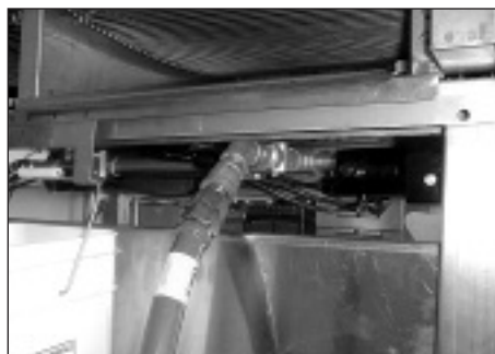
N524/550 Equipment Side Gas Connection
