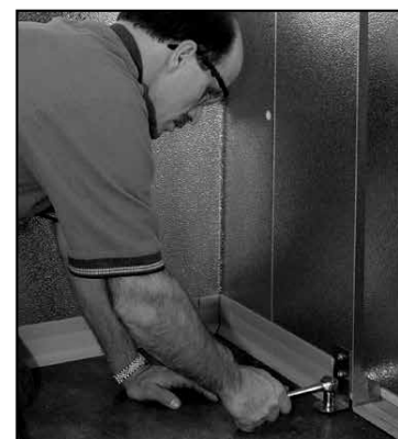
Attach slam brace with fastener provided
