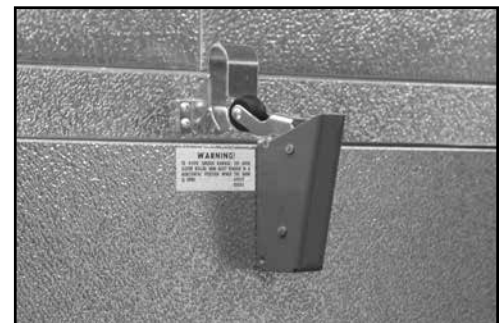
Roller Too High
