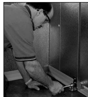
Attach slam brace with fastener provided
