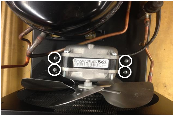
Figure 6-10. Fan Mounting Hardware
