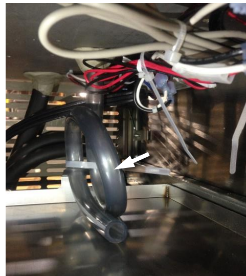
Figure 6-3. Evaporator Condensate Trap
