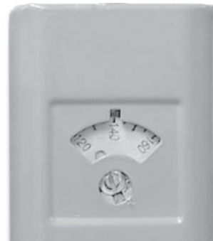
Figure 1. Tankstat Adjustment
