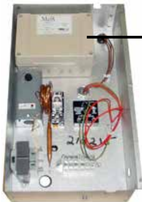
FIGURE 26 - AquaSaver Microprocessor Control, P/N 205044, in the Junction Box
