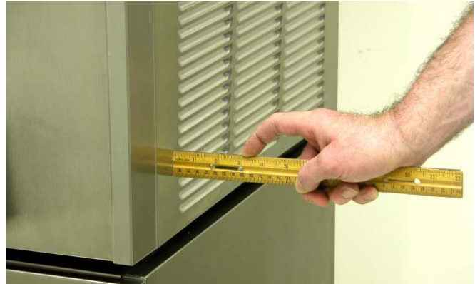
Figure 2-2 Space and Ventilation Requirements
