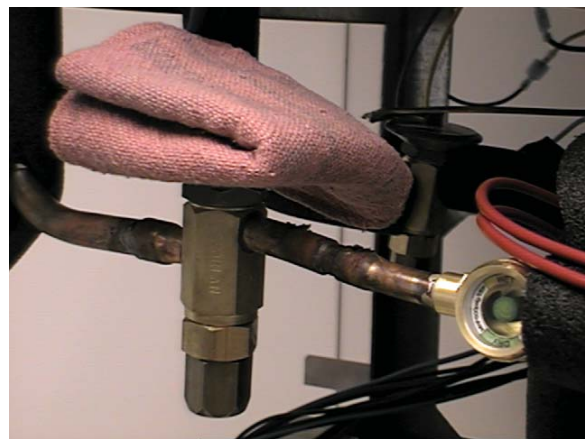
Figure 2-5 TXV Removal
