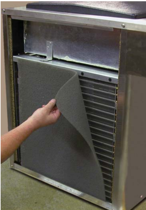
Figure 3-11 F112 Condenser Filter Removal
