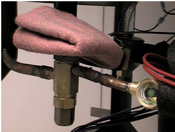
Figure 5-5 AXV Removal
