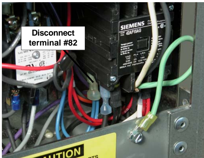
Figure 5-2 Disconnect Compressor Coil
