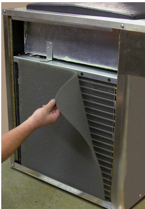
Figure 3-11 F112 Condenser Filter Removal
