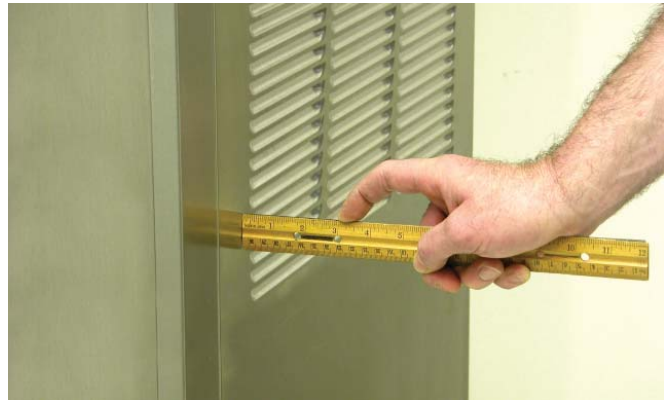
Figure 2-1 Space and Ventilation Requirements
