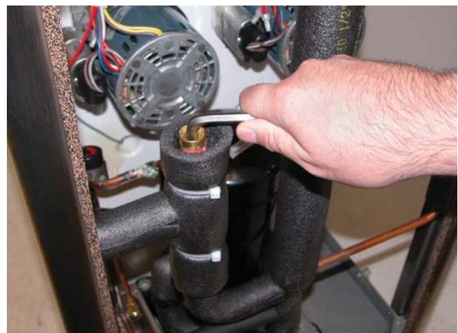
Figure 5-10 Hot Gas Bypass Adjustment
