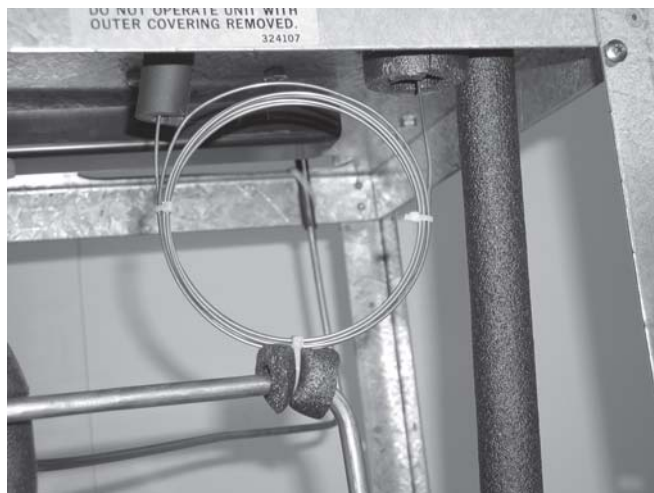
Figure 23. Drier Cap. Tube Assembly
