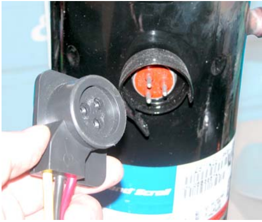
Figure 5-3 Compressor Connection
