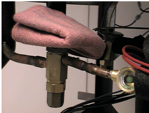
Figure 5-5 TXV Removal
