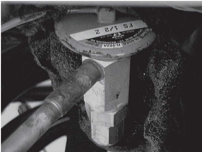
Figure 41. Expansion Valve
