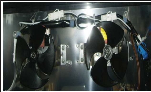
B.Disassemble the evaporator fan motor
