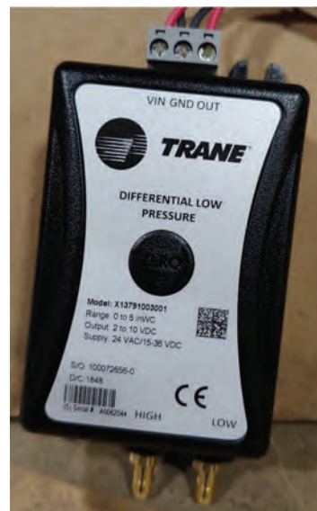
Figure 162. Typical transmitter install for DDP fans
