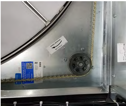
Figure 164. Confirm proper belt tracking on wheel rim
