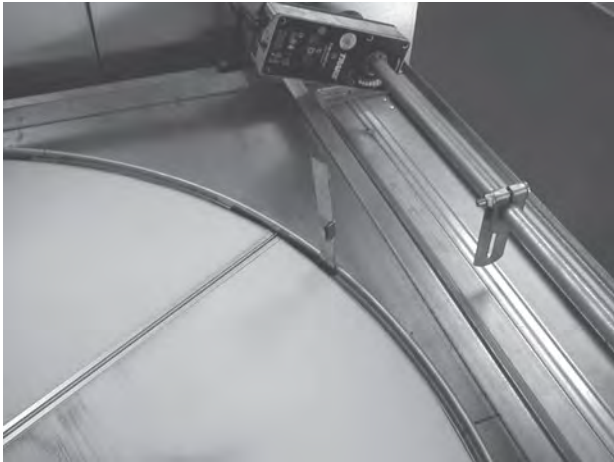
Figure 163. Completely fasten segment retainers
