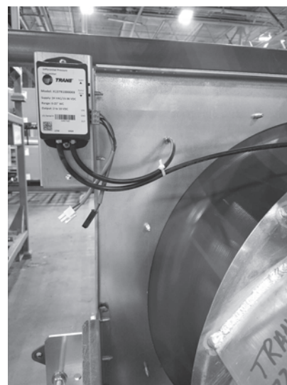
Figure 162. Typical transmitter install for DDP fans
