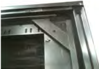
Figure 29. Coil structural gusset
