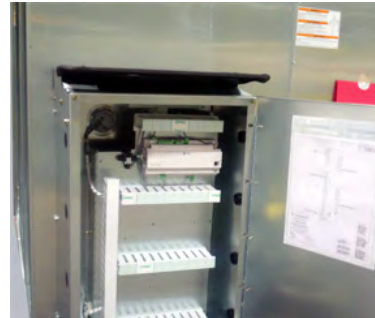
Figure 145. Externally mounted control box
