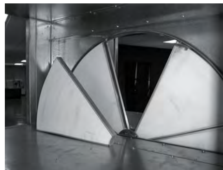
Figure 187. Pull the segment up and out of the wheel frame to remove
