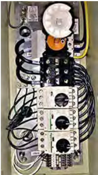
Figure 142. External motorized impeller control panel (MICP)
