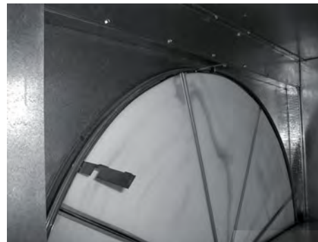
Figure 187. Pull the segment up and out of the wheel frame to remove
