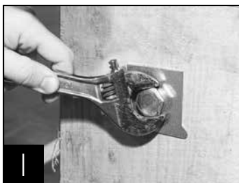
1 Removing skid from bottom of cabinet.
