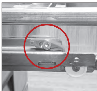
Fig. 5. Drawer retainer location. Retainer is engaged.
