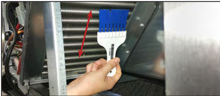
Fig. 3. Never brush across the coil fins.
