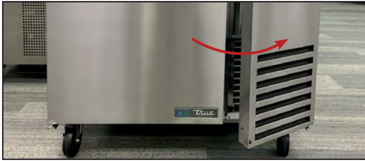
Fig. 1. Open the grill assembly door (TPP & TUC/TWT-44/67/93).
