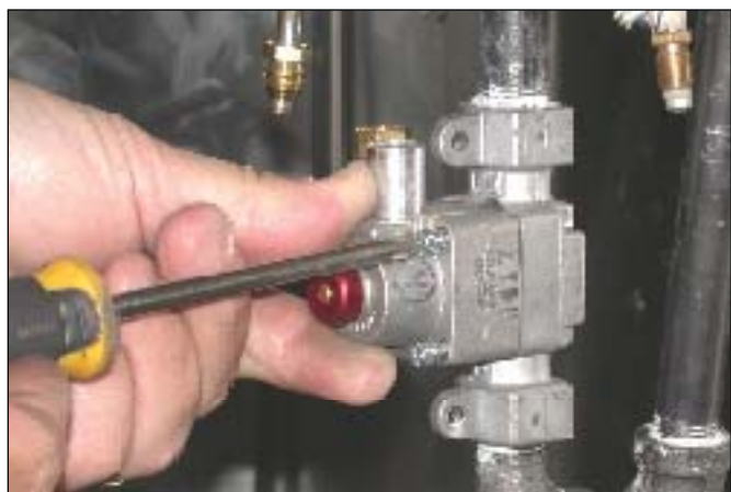
3 Remove the screws from the safety head
