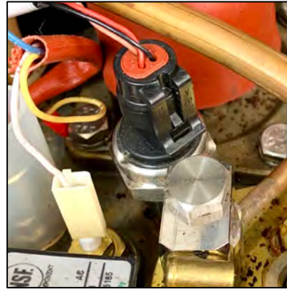
Controlled by Pressure Sensor (Transducer)
